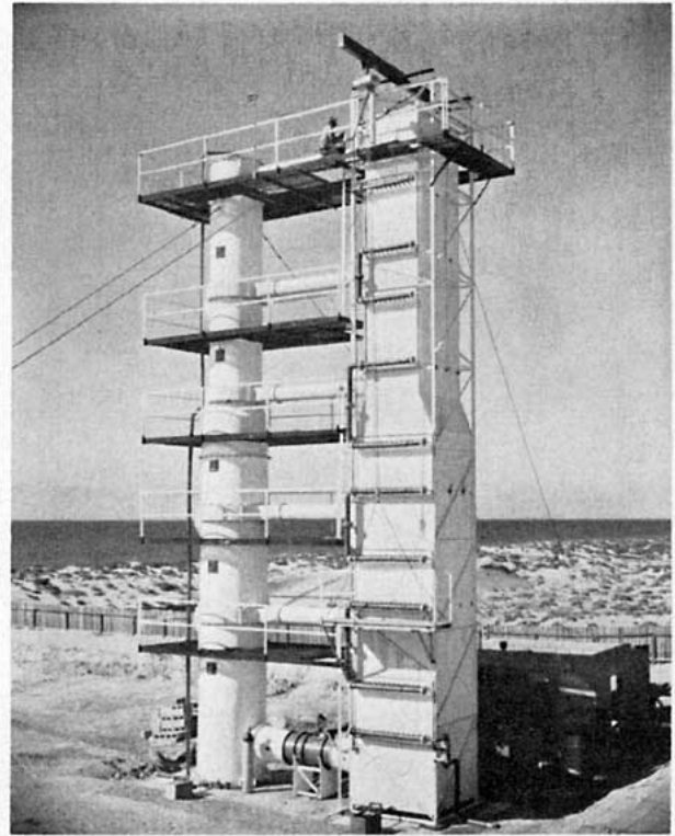
FIG. 3. The evaporator (left) and condenser (right) components of the Puerto Peñasco solar desalination plant. The Gulf of California is in the background.
