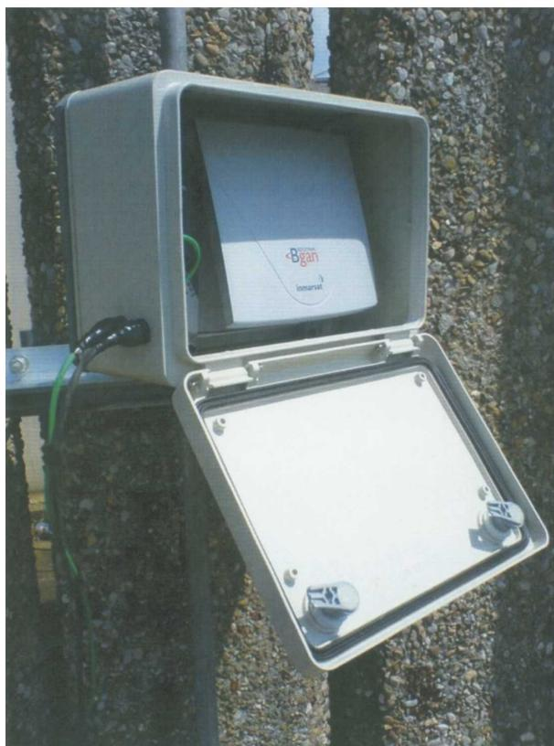
FIG. 2. (a) A radar tide gauge installed at Liverpool communicating via an Inmarsat RBGAN or BGAN terminal. (b) The terminal can be mounted on a nearby post or wall and is approximately the size of a laptop computer.
