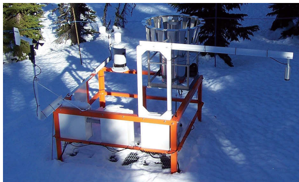
FIG. 2. Custom automatic winter weather stations, such as this, were built to meet the needs of the specialized conditions in a coastal complex terrain environment. They have been placed in both valley and slope-side locations. The photo shows a high-capacity snow gauge, an acoustic snow-depth sensor, a temperature/presure/humidity unit, solar panels, wind sensor, cellular internet protocol antenna, and data logger.
