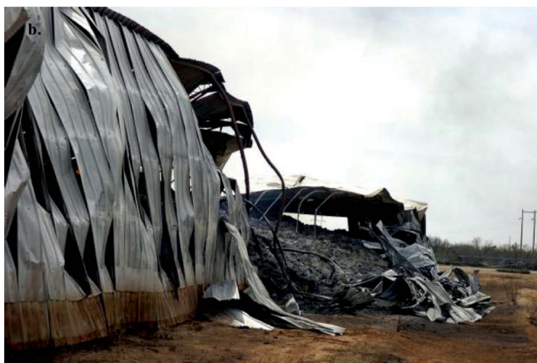
FIG. 1. (a) Home and property destruction near Archer City, TX. (b) Steel-framed storage barn destroyed near Electra, TX. Note that the heat of the fire has deformed the metal frame. Photographs courtesy of the 10 Apr 2009 edition of the Times-Record News of Wichita Falls, TX.
