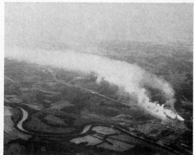
FIG. 2. Wet cooling tower and dry flue-gas plumes from the Paradise Steam Plant (T.V.A.). Although this enlarged photograph lacks background definition, it is useful in illustrating the difference between wet and dry plume behavior in a conditionally unstable environment.
