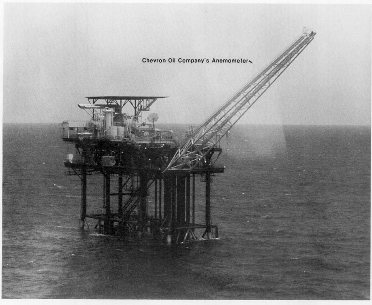
FIG. 2. Chevron Oil Company's Garden Banks 236A gas production platform. The photo was taken prior to installation of the C-MAN measurement equipment, including a 6.1-m mast and anemometers near the end of the boom.
