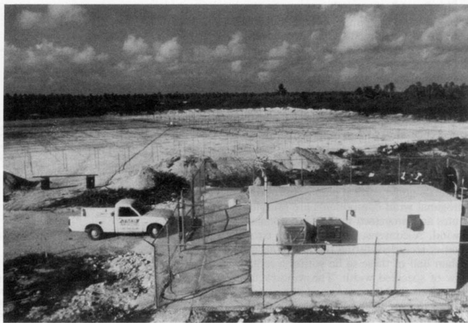
FIG. 2. The Christmas Island wind profiler. Shown is the antenna that comprises a phased array of coaxial-collinear elements and the laboratory building that houses the computer and hardware subsystems.
