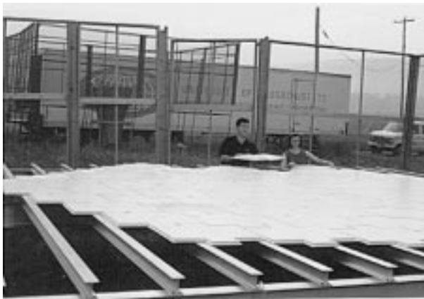
FIG. 4. TEP receive array under construction in the field. Clutter fences, the transmit horn, and the trailer are visible in the background.
