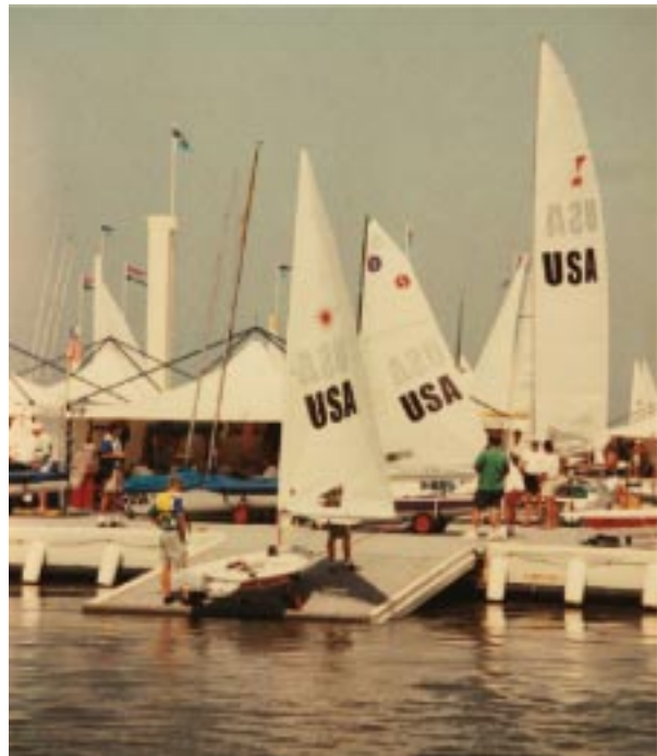
FIG. 8. The day marina was the primary boat launching facility and consisted of several steel barges moored to the bottom by steel columns and covered by all-weather carpet. Athletes were sheltered in tents supported by steel frames.
